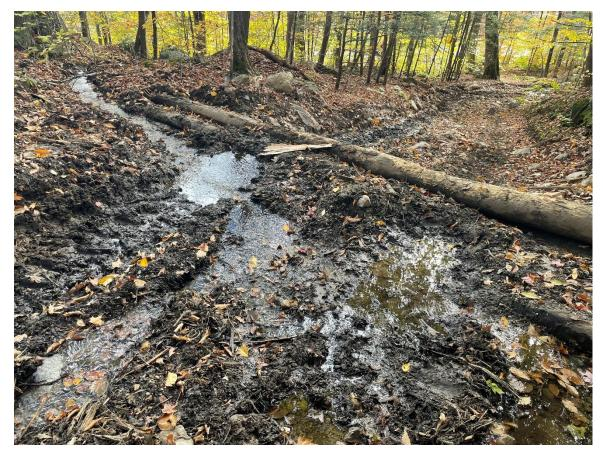
Example of log reinforced water bar on the active harvest. Photo credit: Colin Mettey
